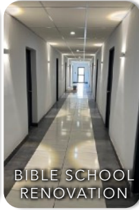
RENOVATION OF BIBLE SCHOOL DORMS
